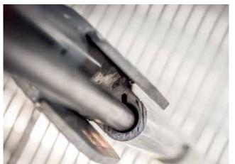
The inner doors have a round hinge profile and rounded sides to prevent injury. The cavity for the steel locking pin is equipped with blind drainage. This ensures proper functioning even during frost.
